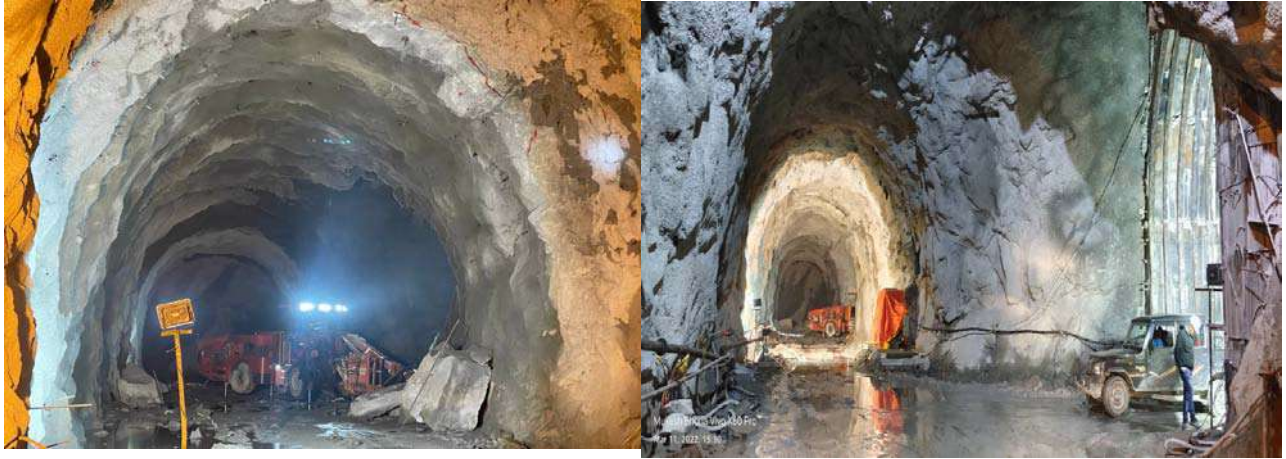
Pressure Shaft Works
