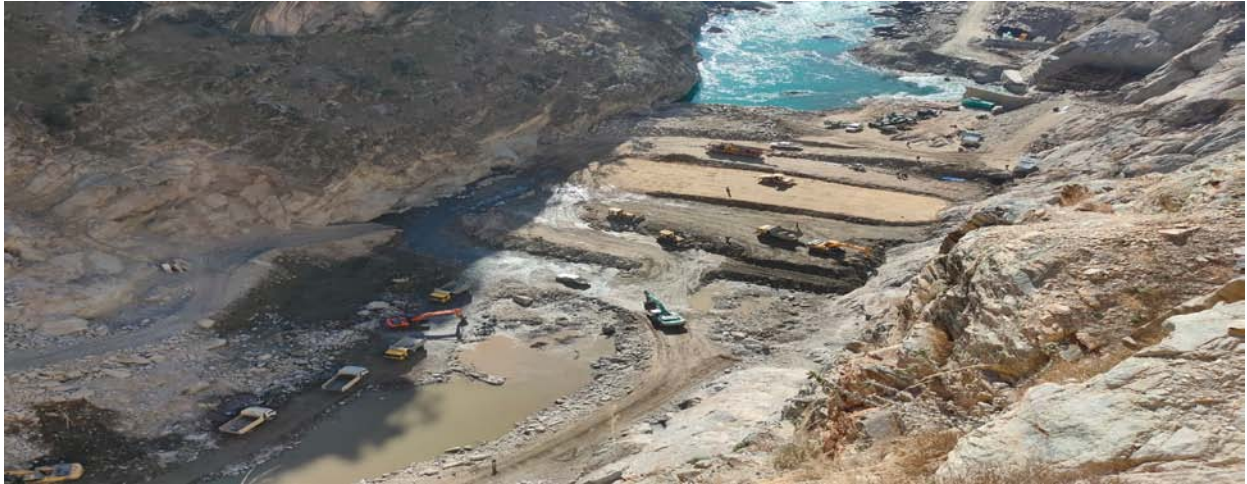
COFFER DAM & DAM EXCAVATION
