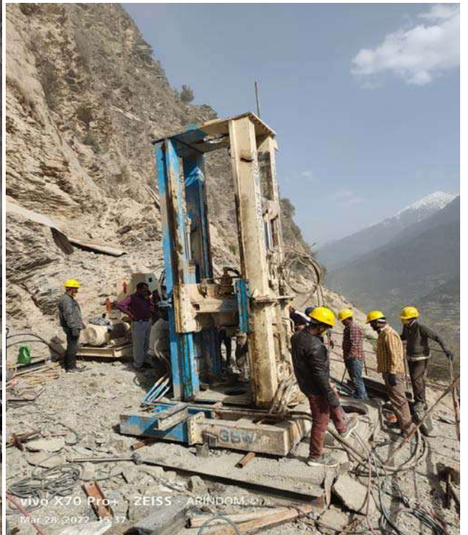
Excavation of Surge Shaft
