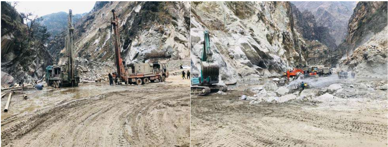
Grouting works are in progress Dam Excavation Below River Bed
