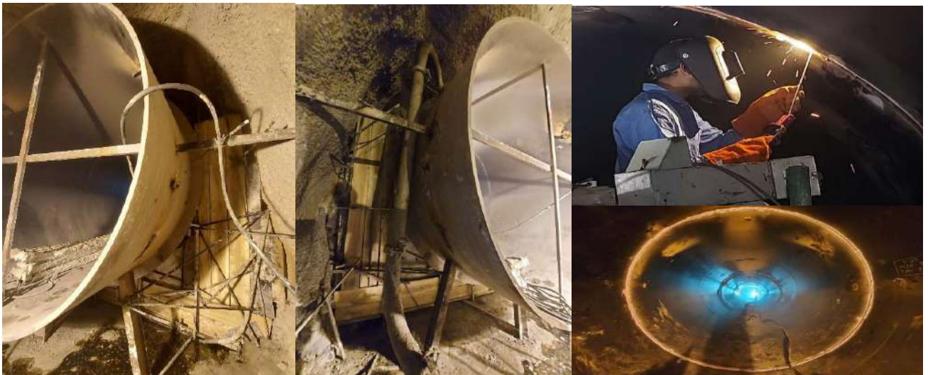
Successful Commencement of Erection of Steel Liner in PS
