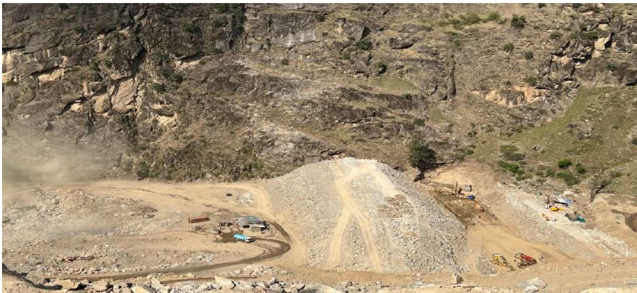
ONGOING CONSTRUCTION WORKS AT UPSTREAM COFFER DAM AFTER RIVER DIVERSION
