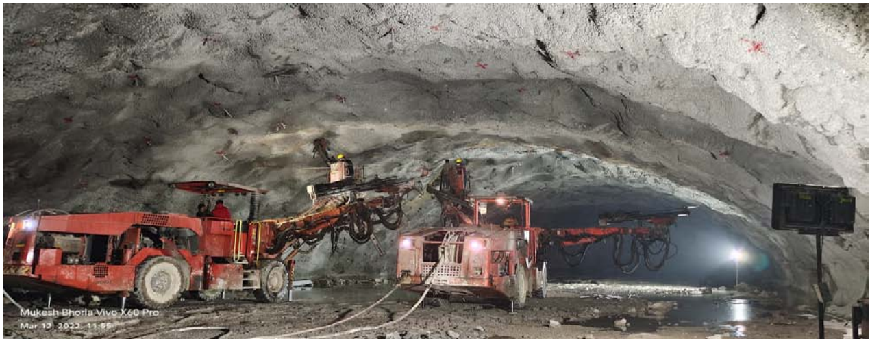
Power House – Crown widening
