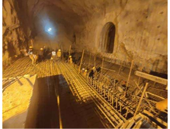
Raft Reinforcement in Transformer Hall Cavern
