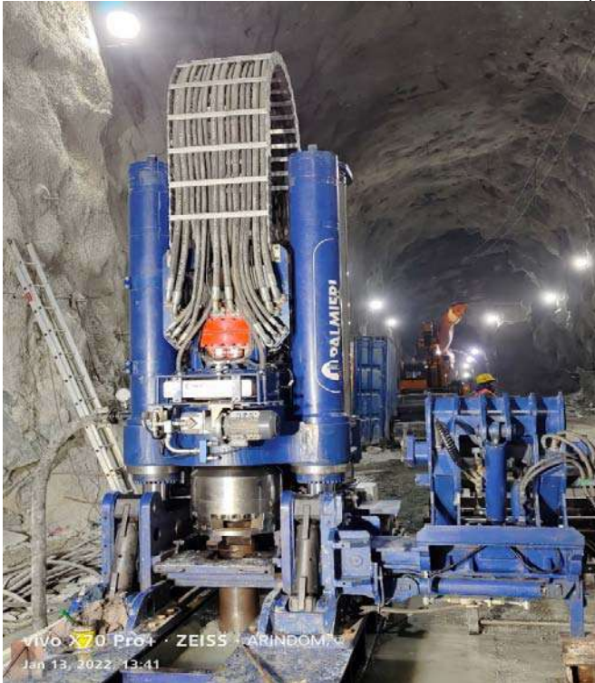
Raise Borer at upper Erection Gallery PS top
