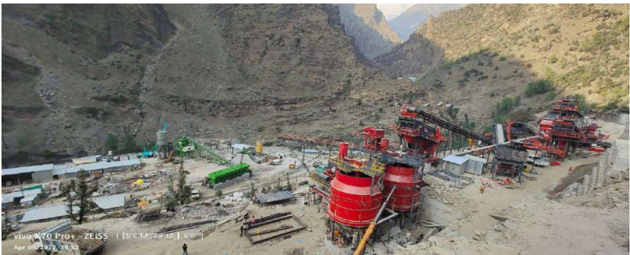
Erection of 600 TPH Crusher Plant
