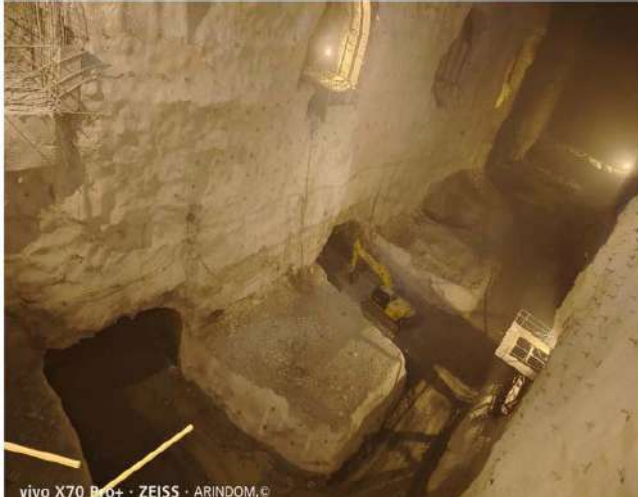
Power House Cavern
