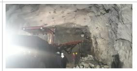
Excavation of Adit from MAT Junction to MIV Chamber Top (159.28m) completed on 05.12.2019
