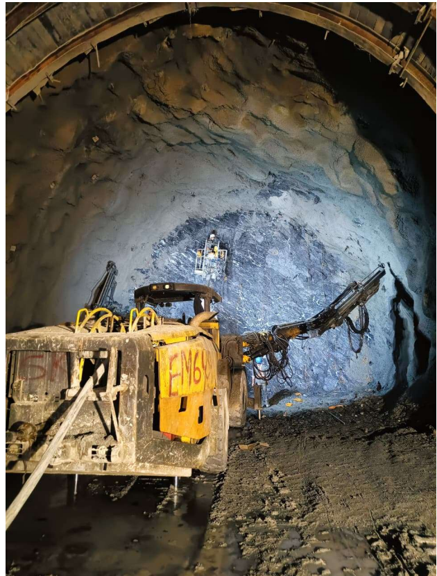
TRT-2 D/S FROM INTERMEDIATE ADIT
