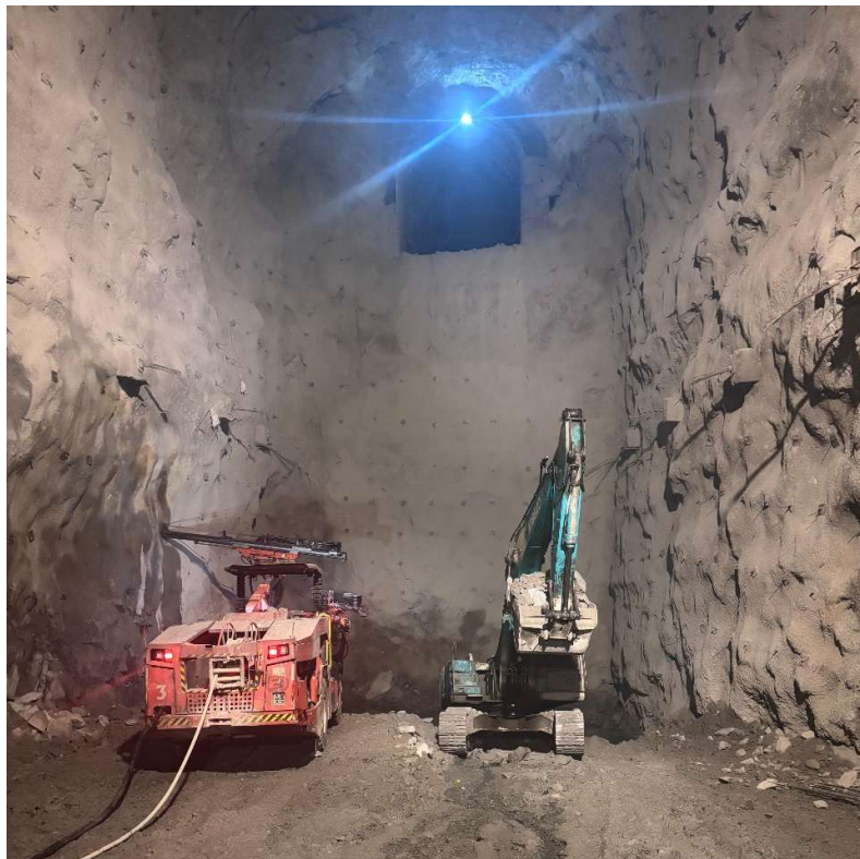
CONTROL BLOCK EXCAVATION
