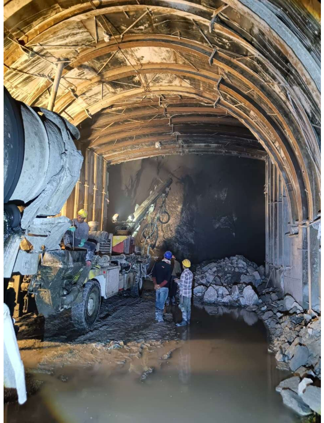
BRANCH TUNNEL LEADING TO DRAFT TUBE#3
