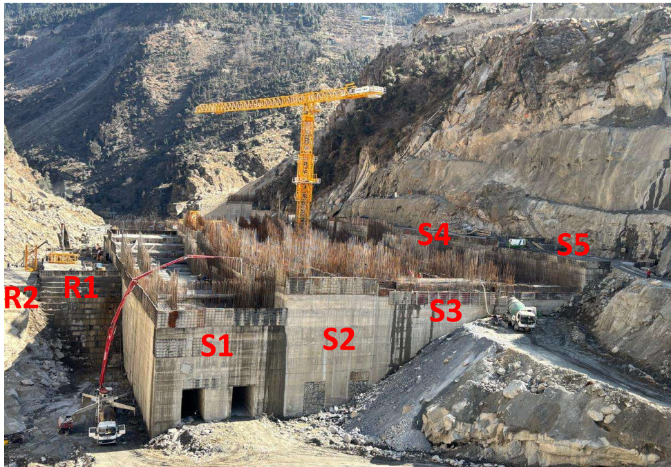
DAM CONCRETING (UPSTREAM AND DOWNSTREAM VIEWS)
