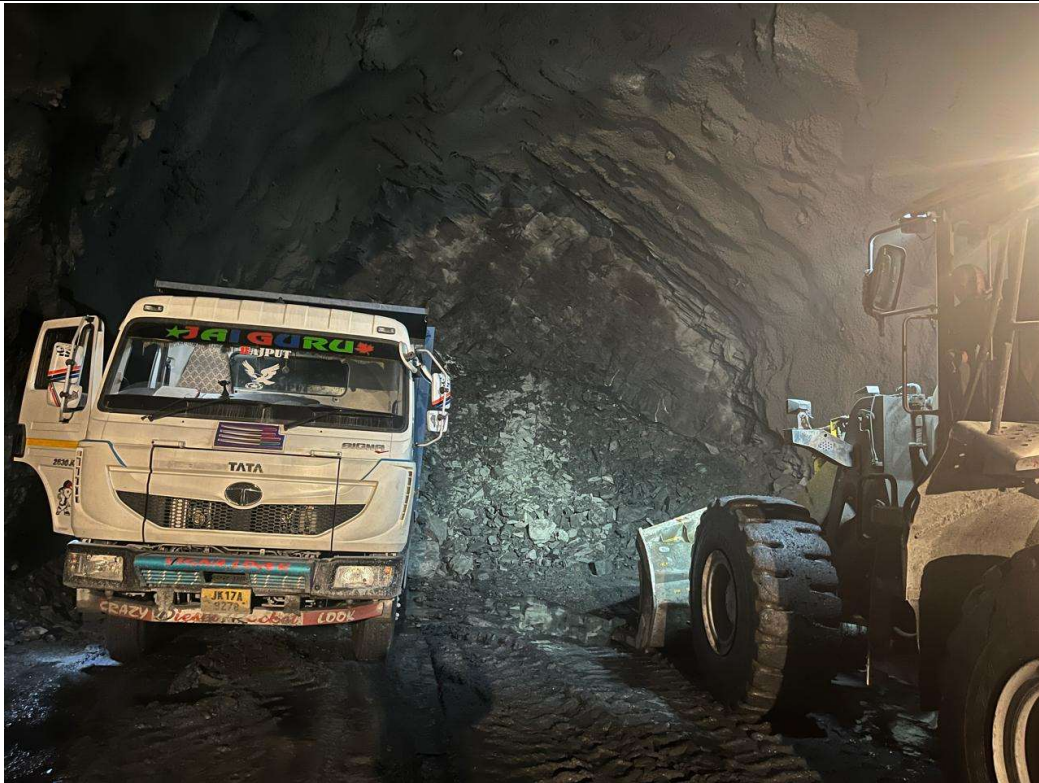
TRT-1 D/S FROM INTERMEDIATE ADIT
