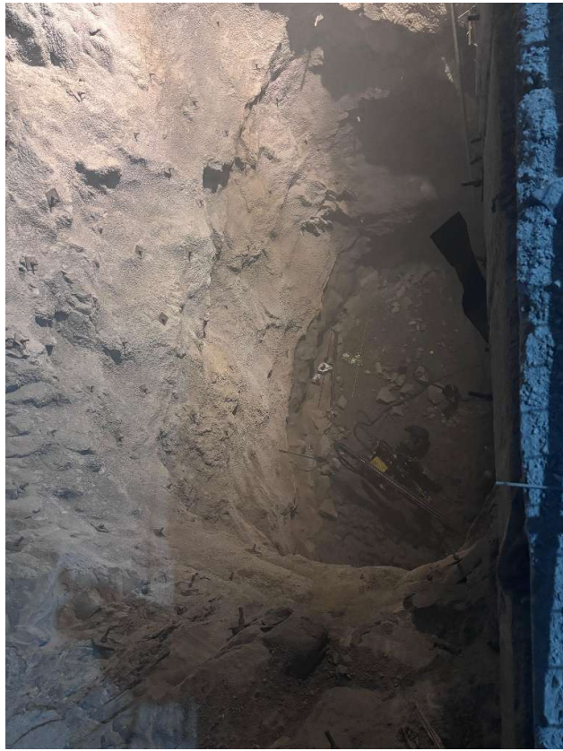
DRAFT TUBE GATE SHAFT EXCAVATION
