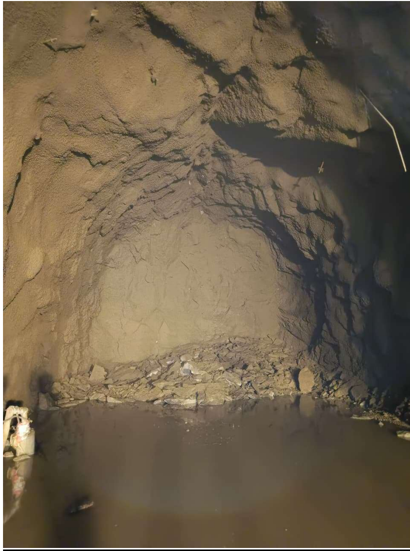
ADIT TO PS BOTTOM
