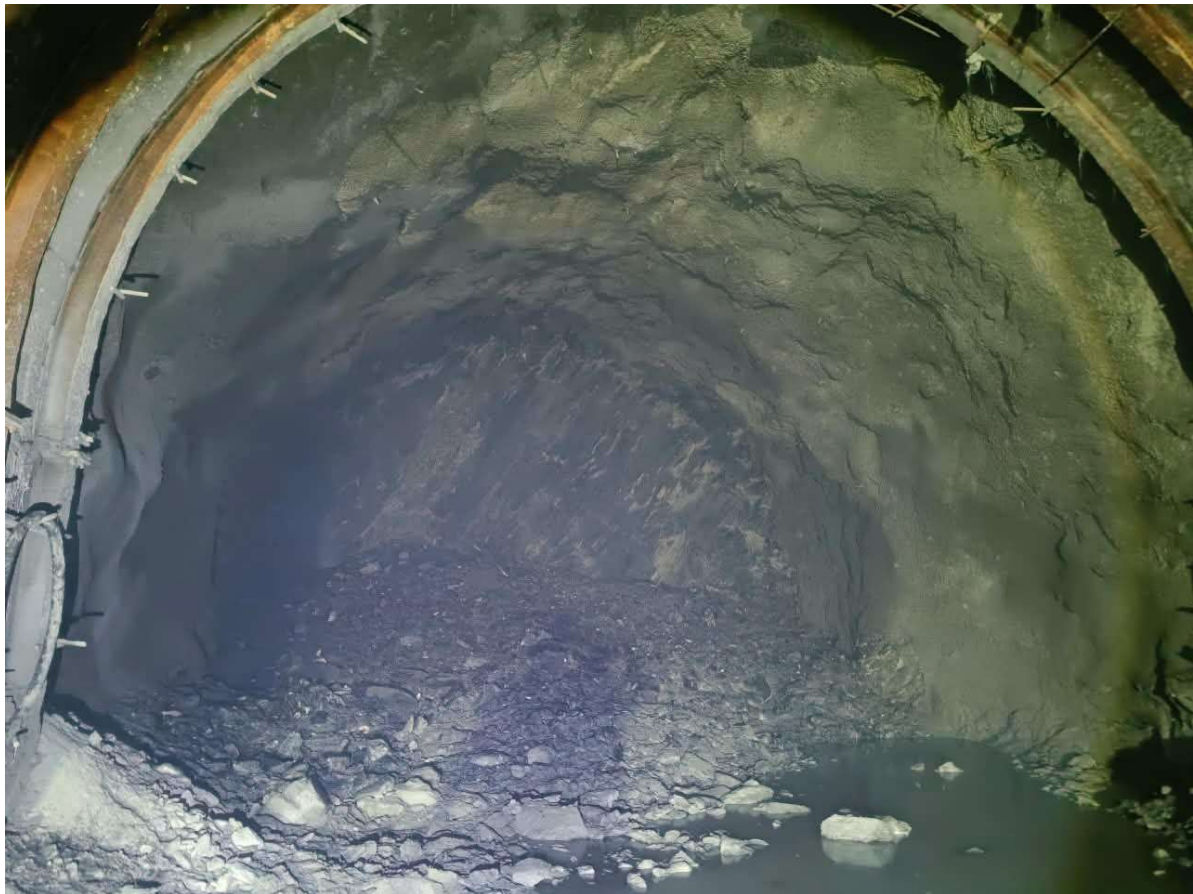
TRT-2 U/S FROM INTERMEDIATE ADIT
