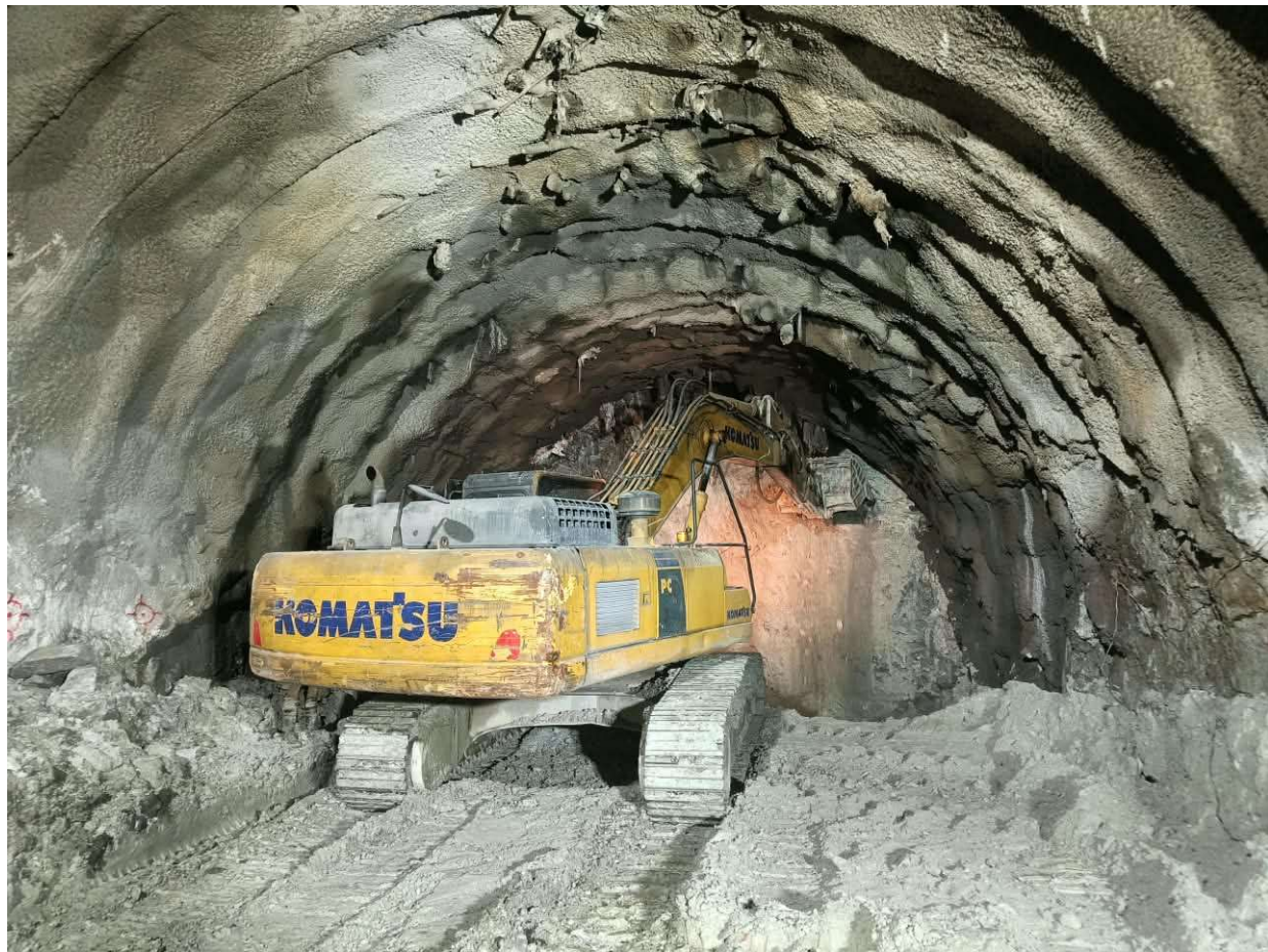
TRT-1 D/S FROM SURGE GALLERY
