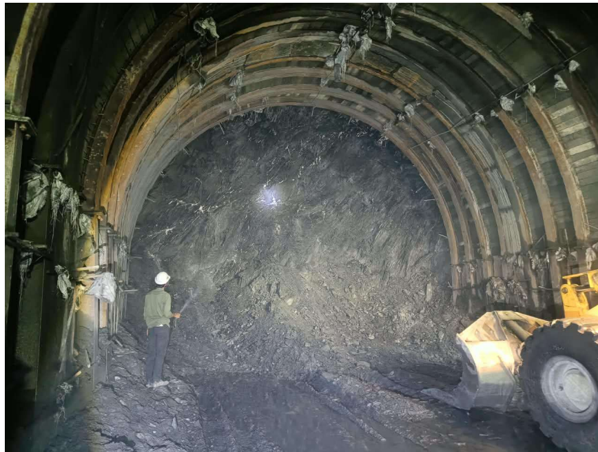
TRT-1 U/S FROM INTERMEDIATE ADIT
