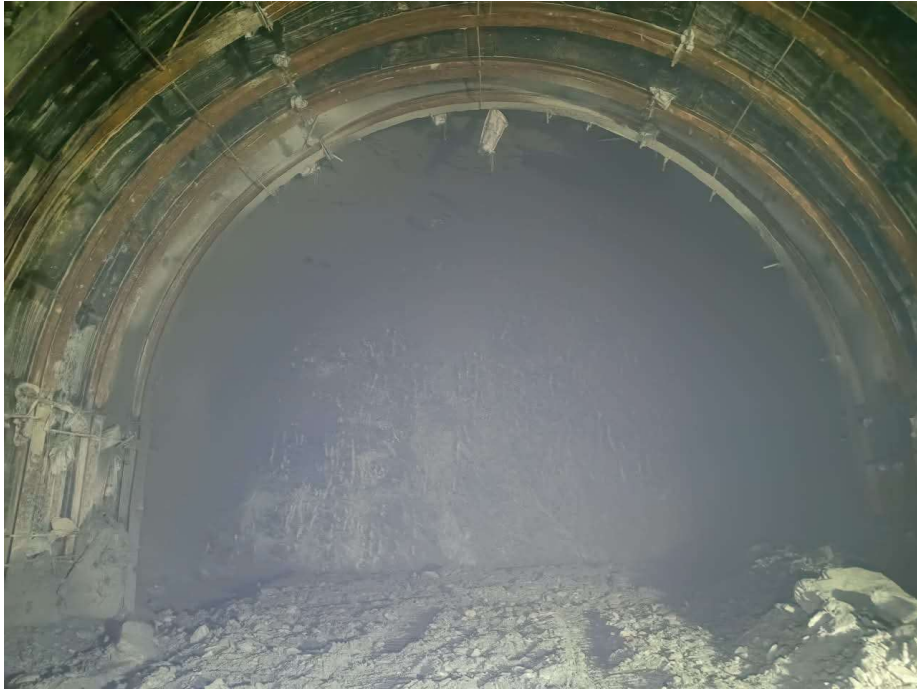
TRT-2 D/S FROM INTERMEDIATE ADIT
