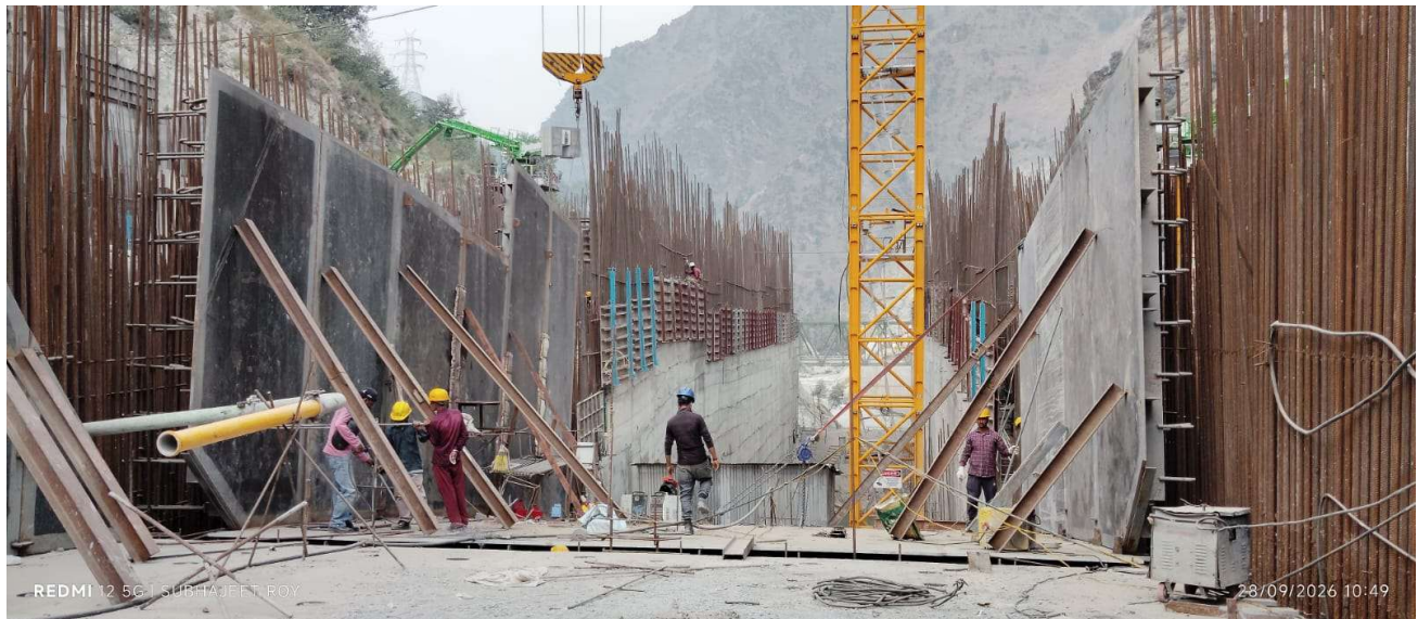
HM WORKS - SPILLWAY SIDE LINERS IN S3 & S4 BLOCK
