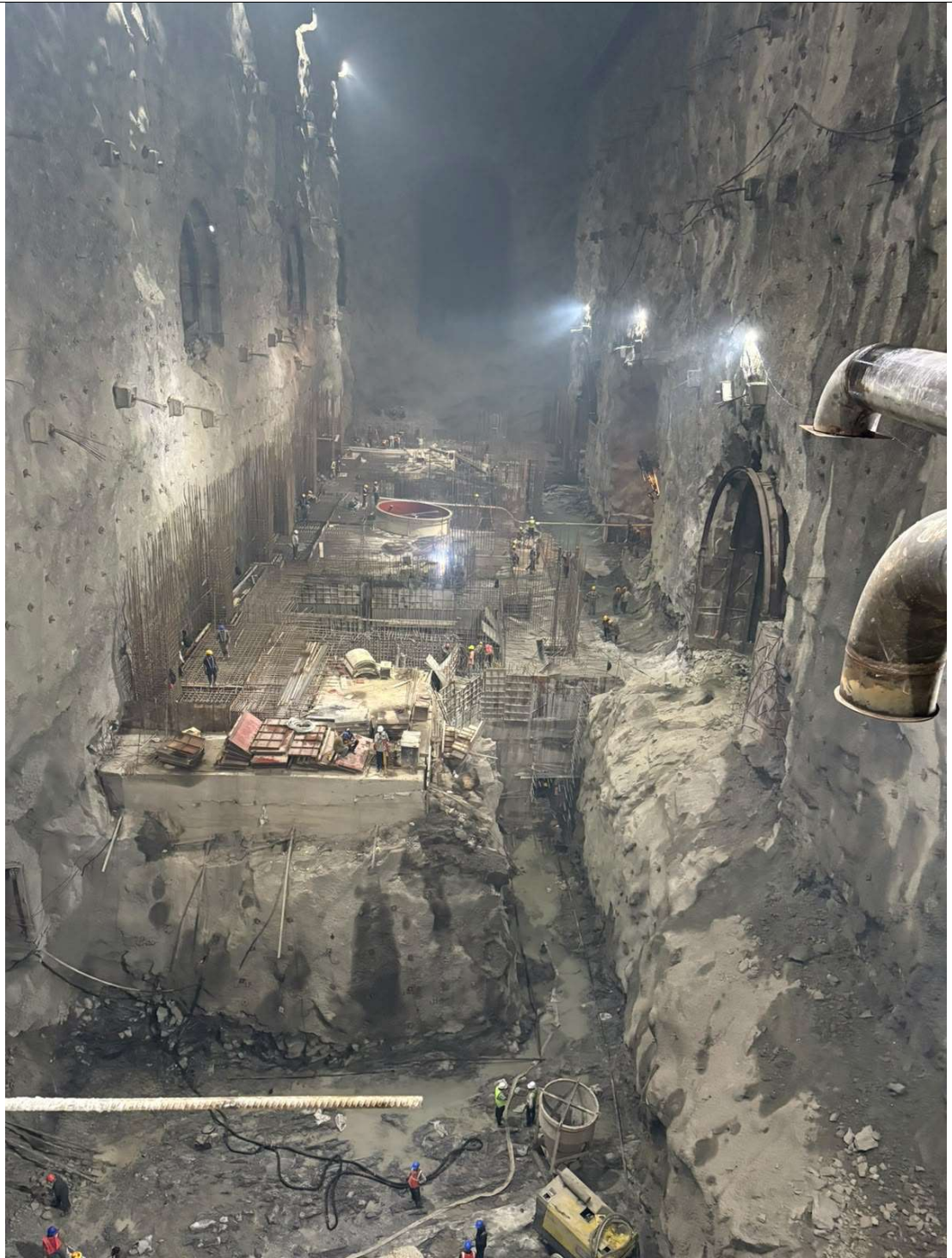
POWER HOUSE EXCAVATION
