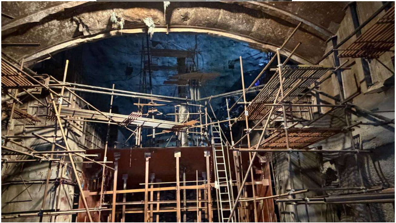
DRAFT TUBE -4 ERECTION
