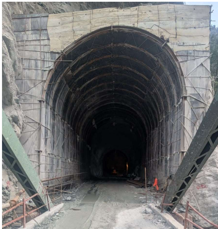
TRT OUTLET WORKS
