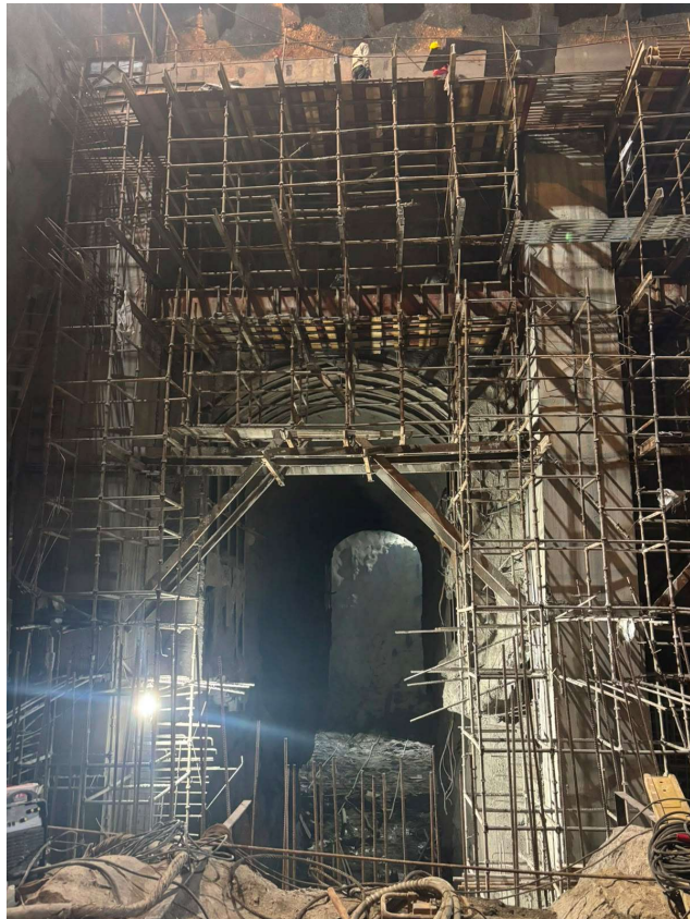
CONCRETING IN SERVICE BAY AREA
