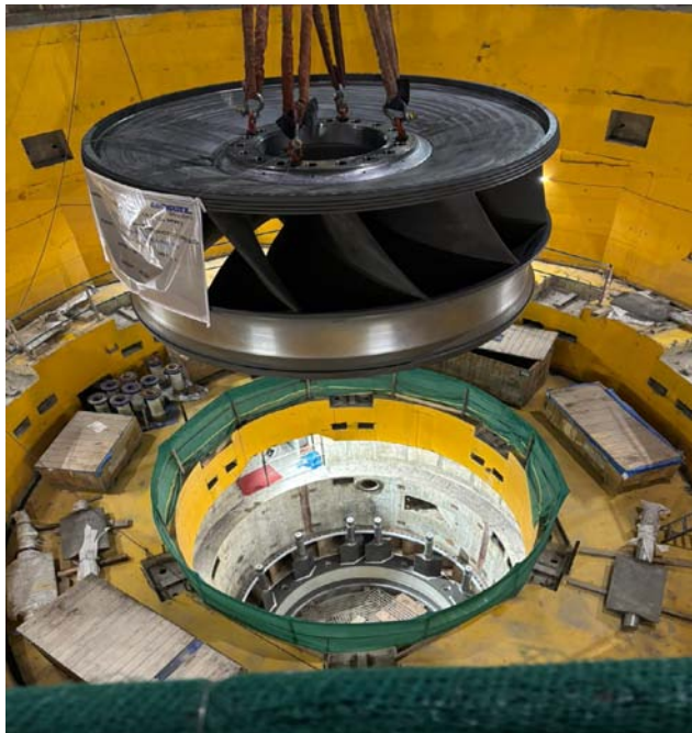
Unit # 1: Lowering of Runner
