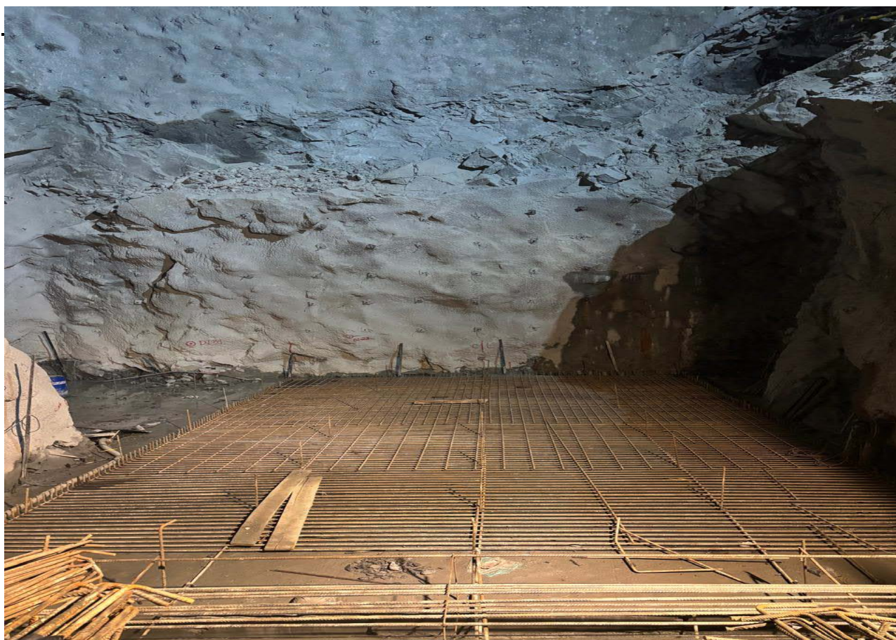
Unit-4 Draft Tube Pit
