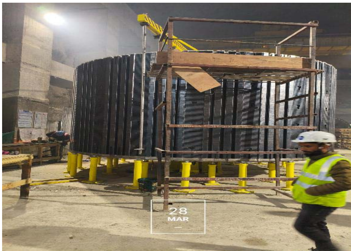
Rotor build-up (Unit-3)
