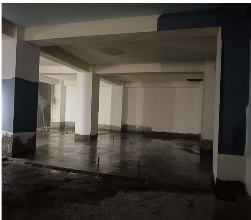
Control Block building Architectural work
