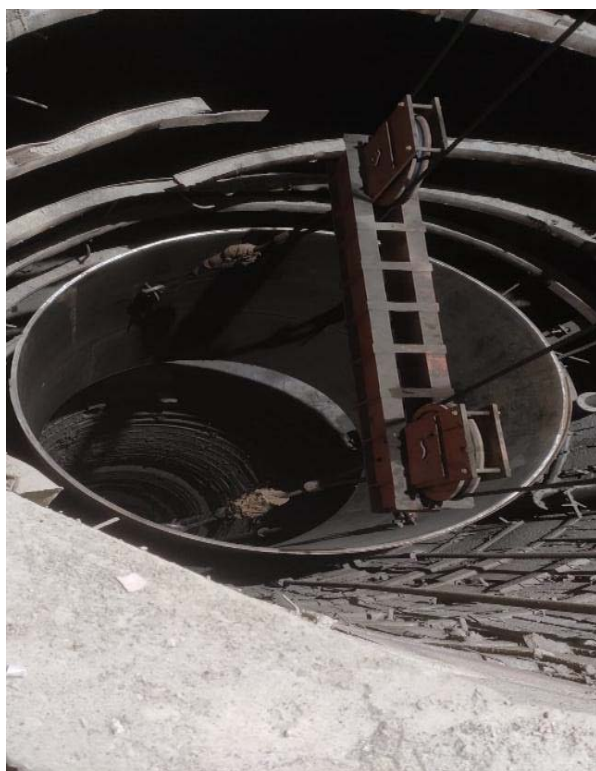
Vertical Pressure Shaft Erection
