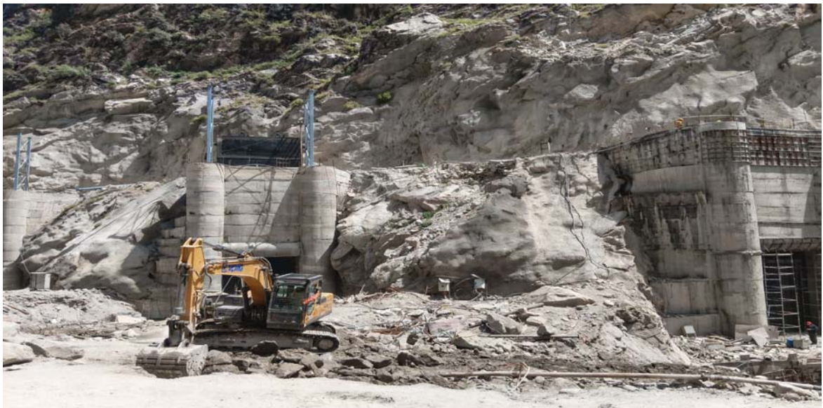
TRT Erection of Gates
