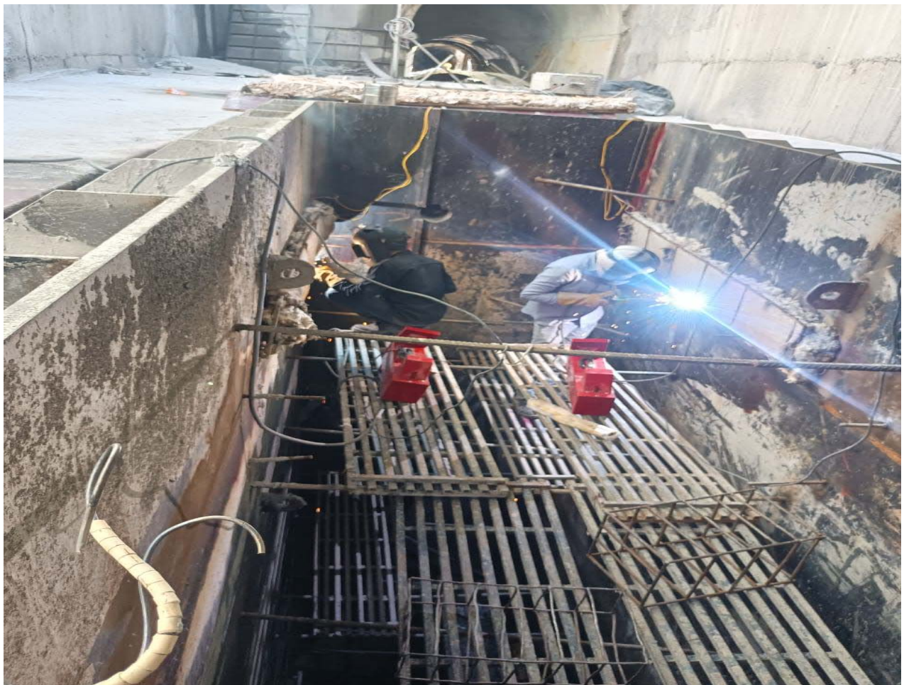
Construction Sluice Steel Liner
