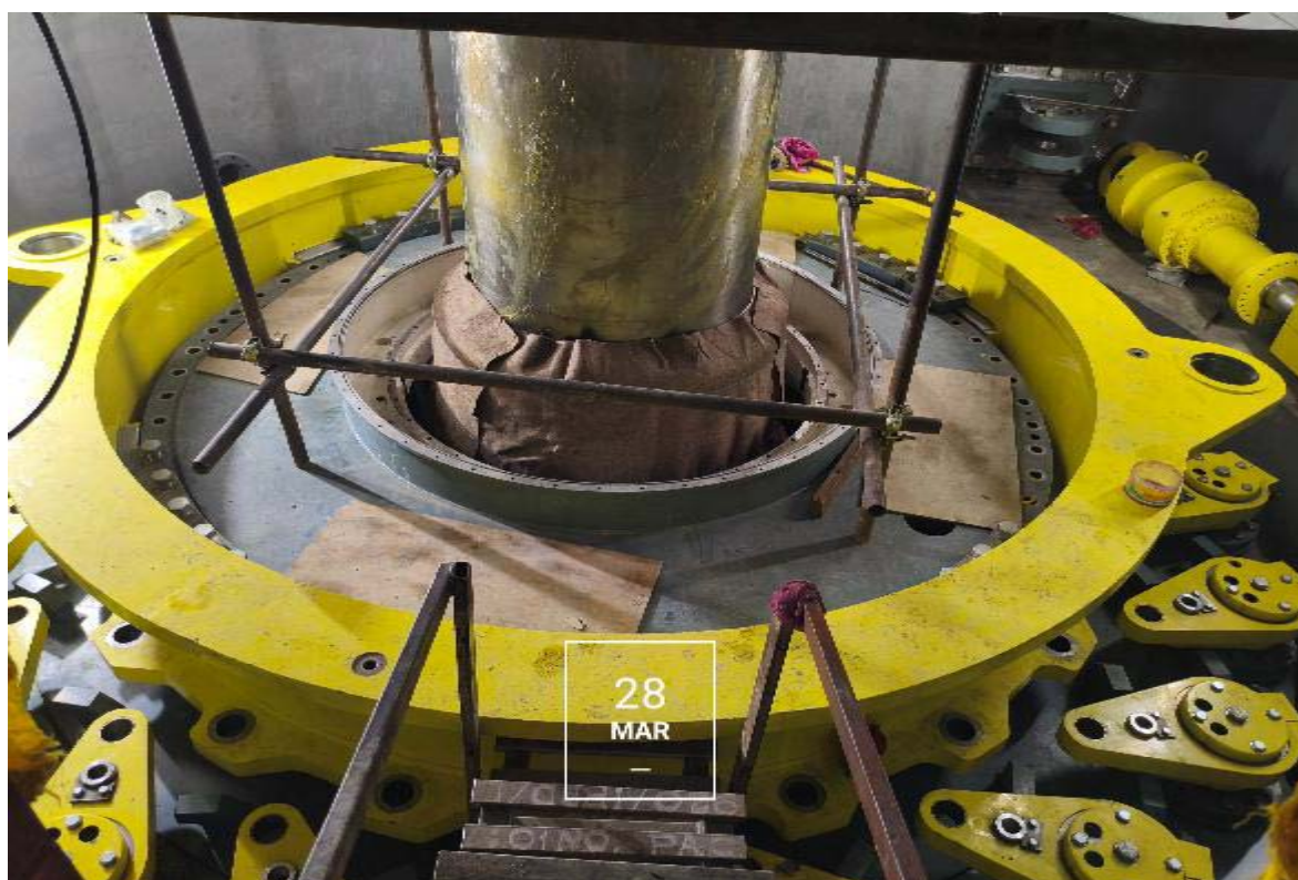
Unit # 3 Installation of Servomotors
