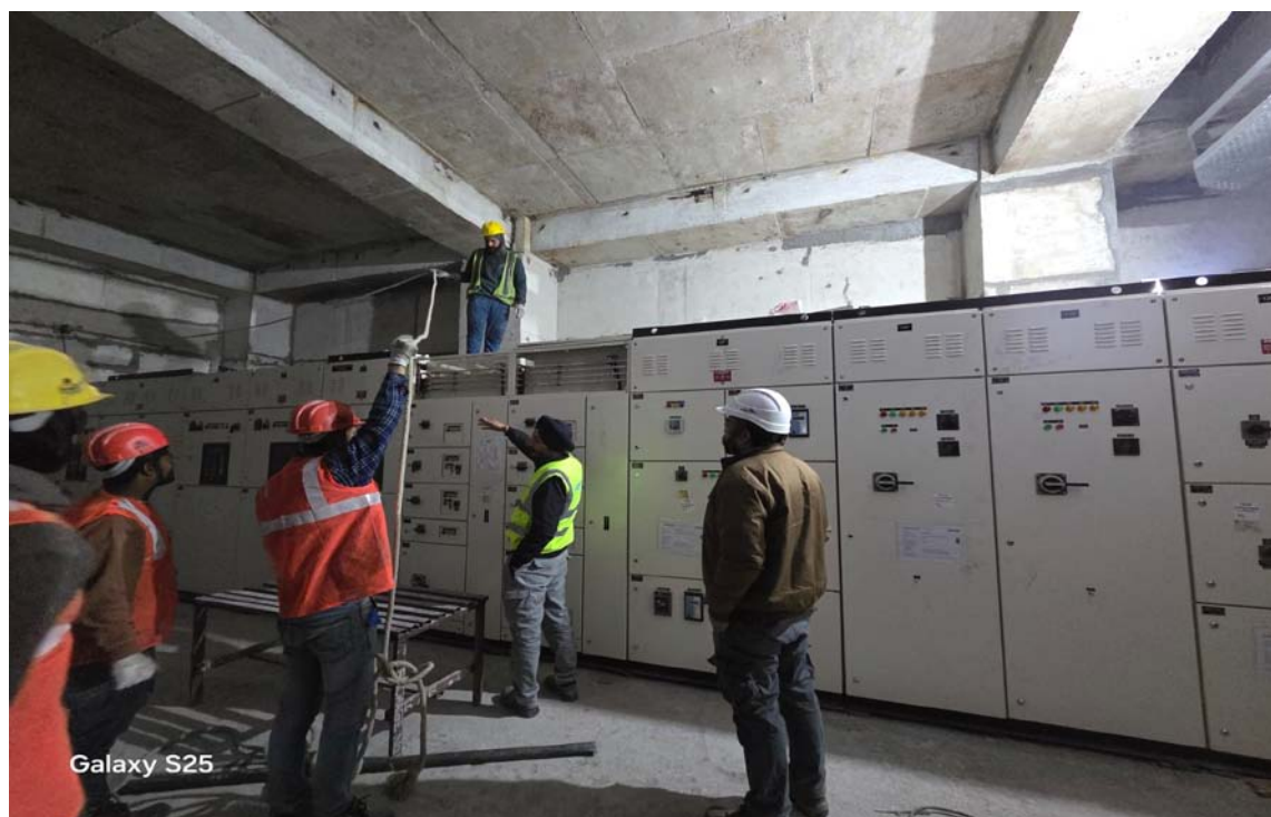
Installation of SSB Panel
