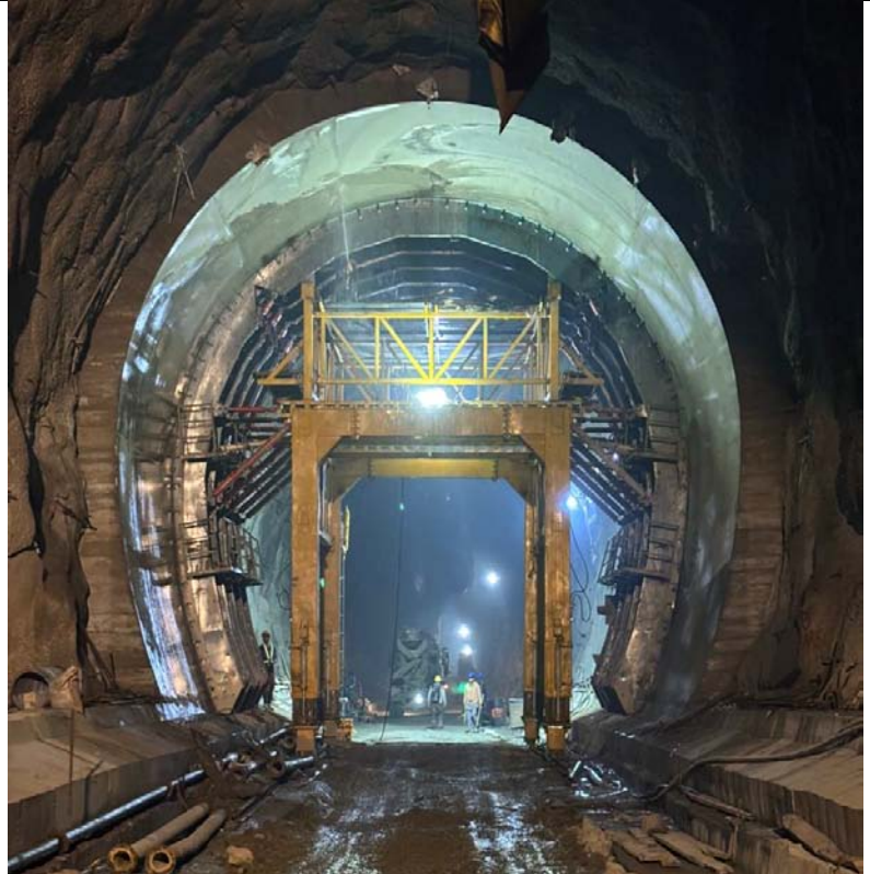
Surge Gallery TRT-2 Lining
