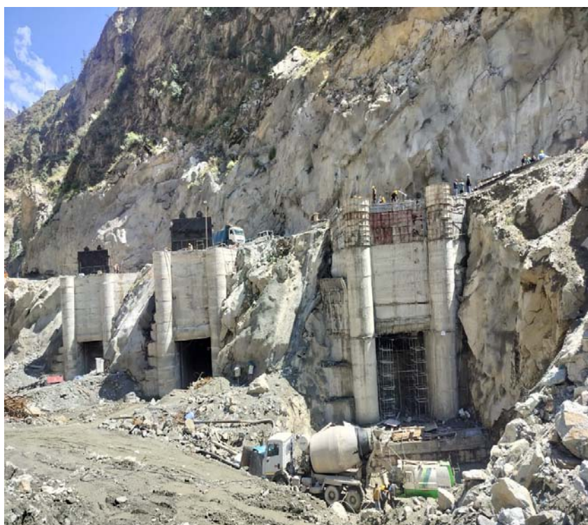
TRT#1, 2 & 3 – Outfall Structure
