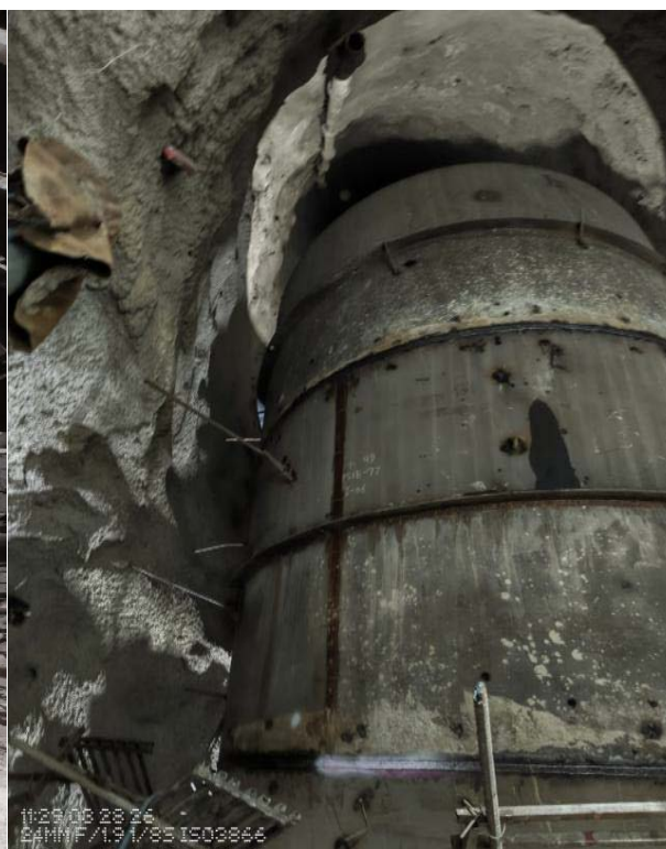
Vertical Pressure Shaft Erection
