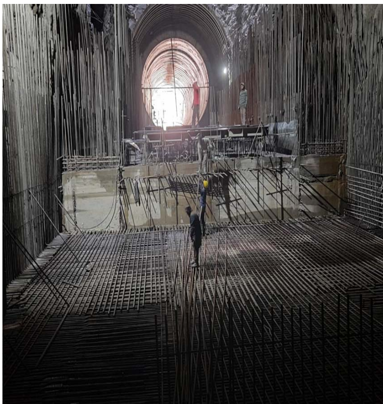
Tunnel Spillway-2 Gate Shaft
