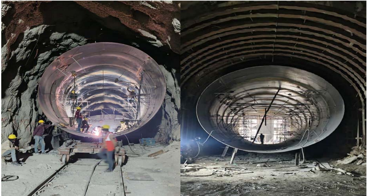
Pressure Shaft Erection of Steel Liners
