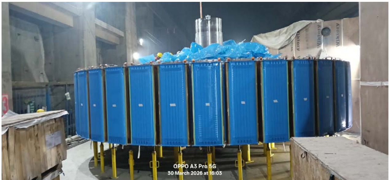
Unit # 1: Rotor Assembly Work
