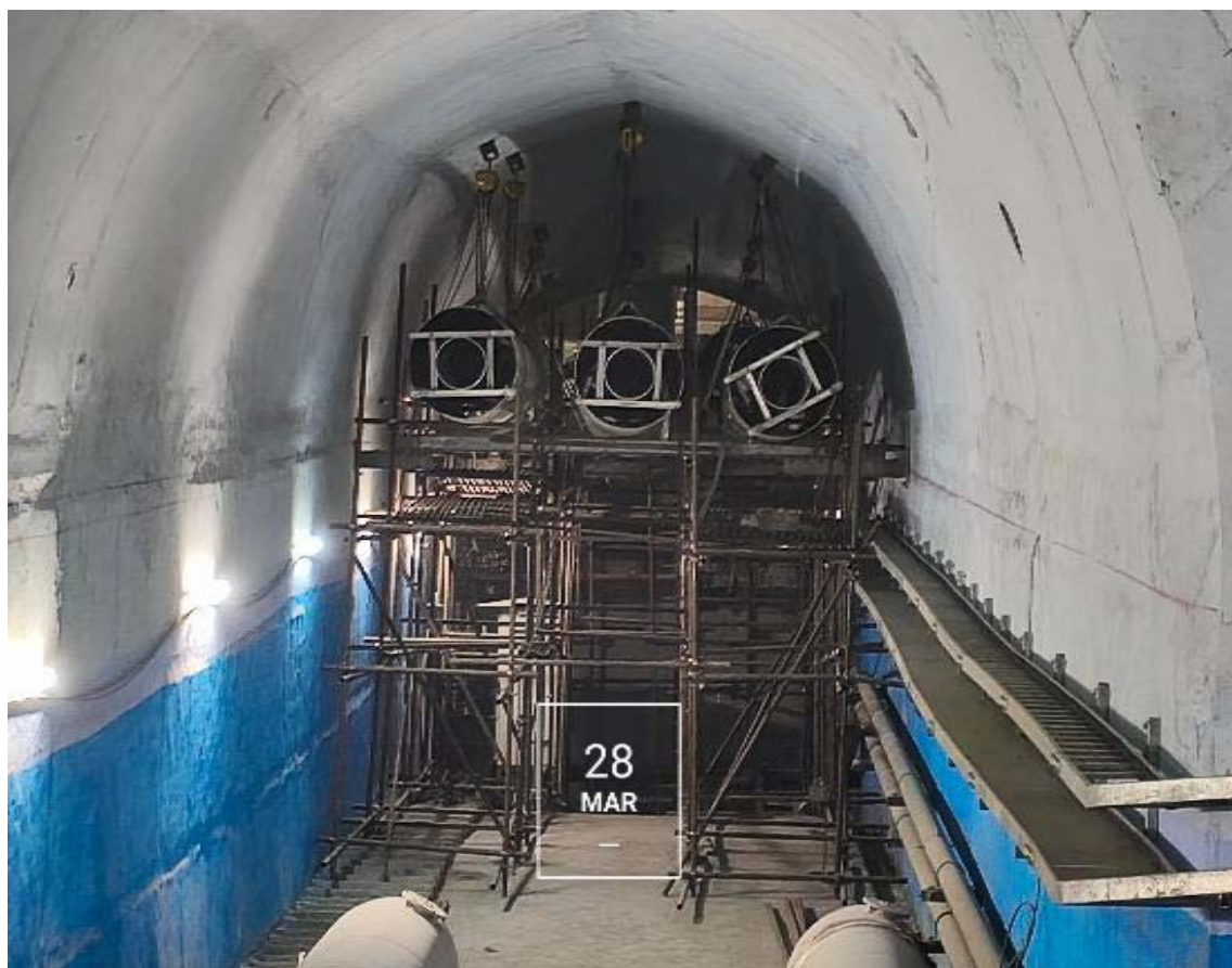
Unit#4 Erection of Bus Duct
