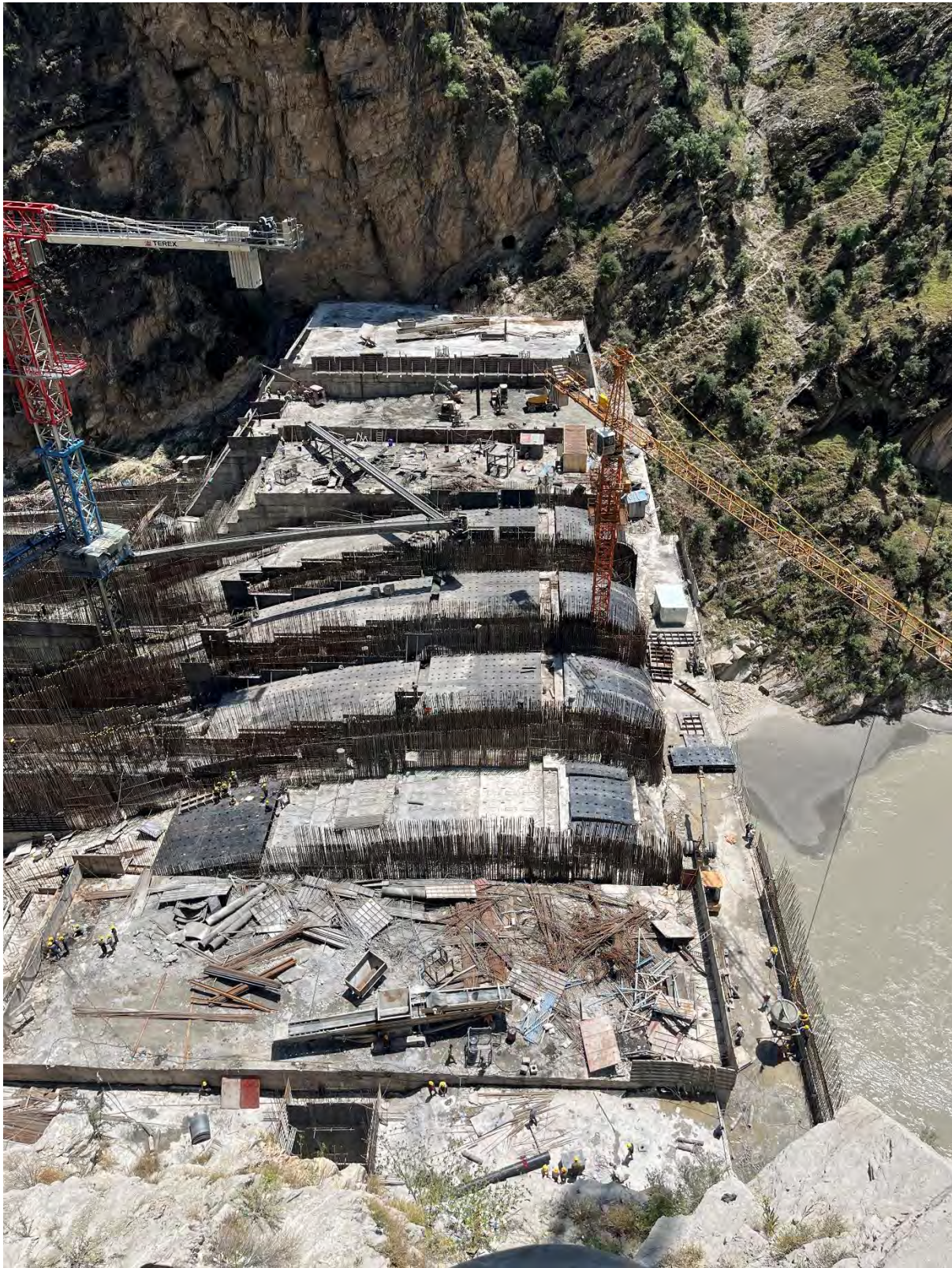
Photo 3. Kiru HEP, Dam construction site.
