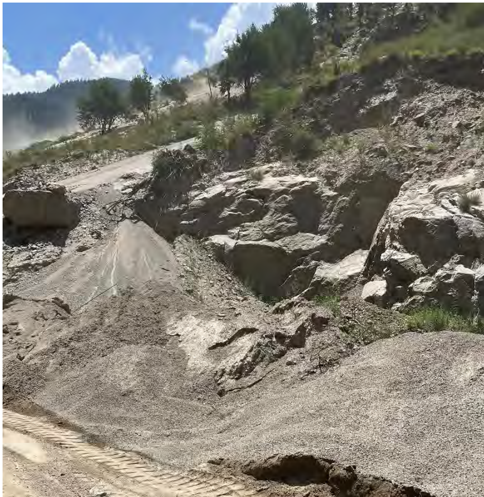
Photo 1. Fugitive emission observed during site visit.
