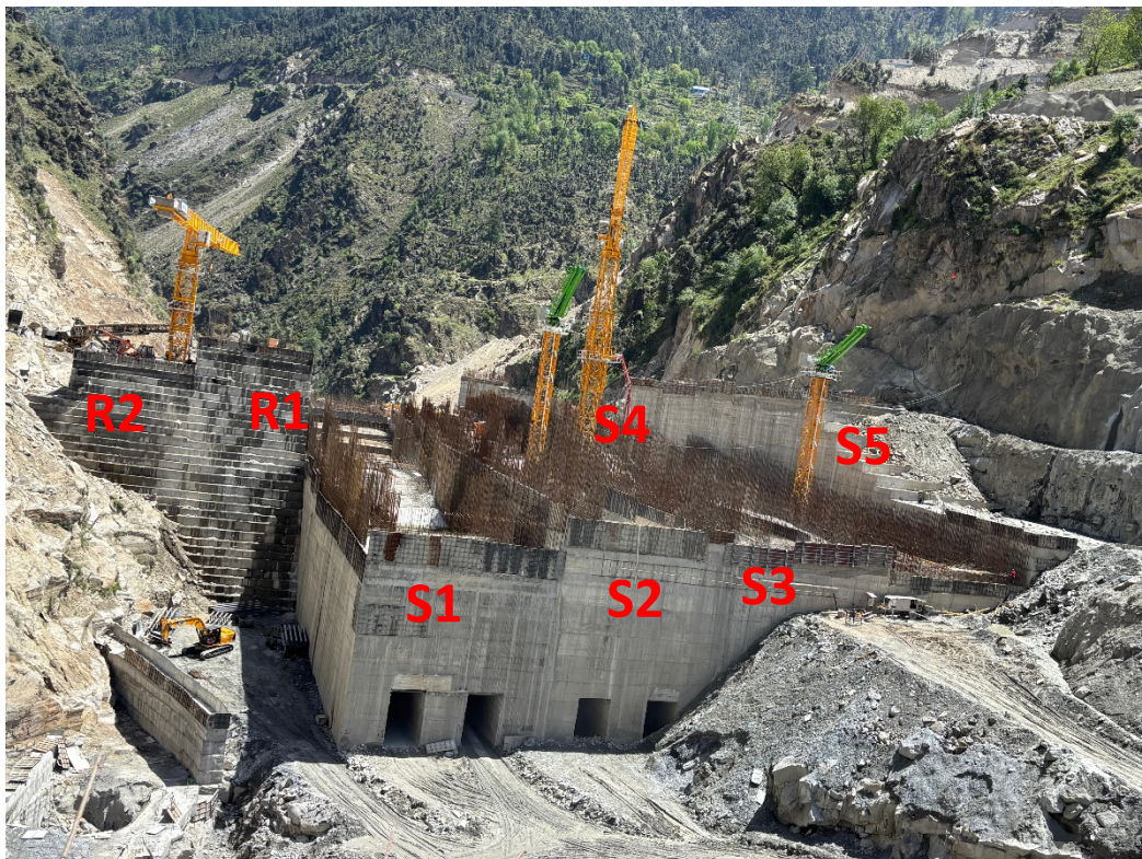
DAM CONCRETING (UPSTREAM AND DOWNSTREAM VIEWS)
