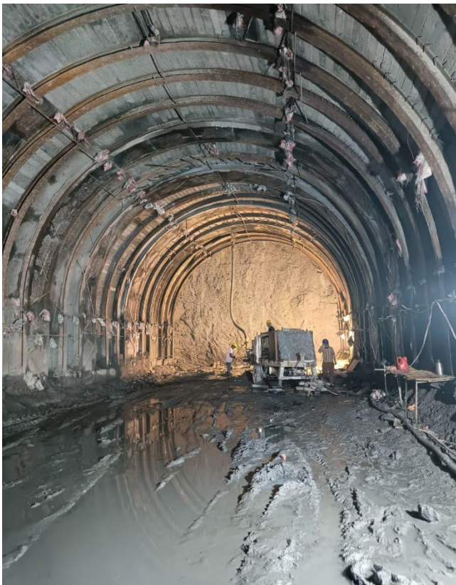
TRT-2 D/s FROM INTERMEDIATE ADIT
