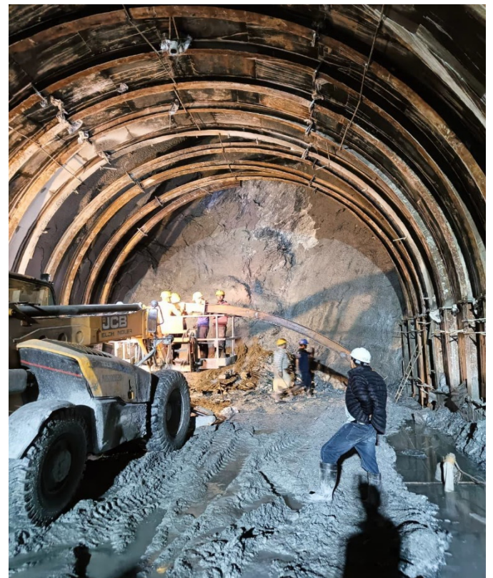
TRT-2 U/s FROM INTERMEDIATE ADIT
