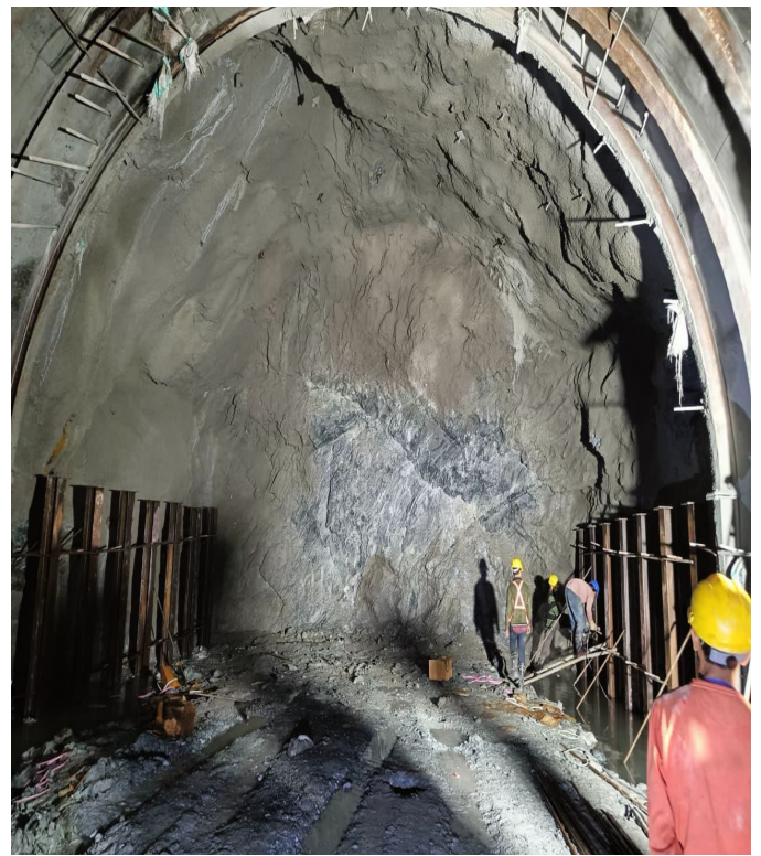
TRT-1 U/s FROM INTERMEDIATE ADIT
