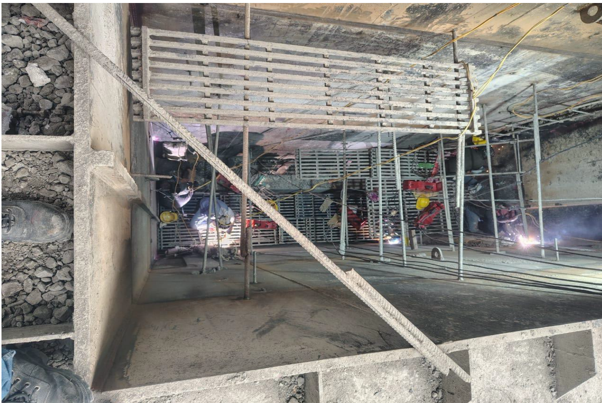
WELDING WORK IN CSG LINER IN S1 & S2 BLOCK
